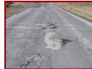
Depicts road failure due to poor soil and topography that cannot be fixed with routine maintenance.
