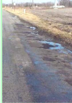
The soil beneath existing roadways is also a major factor in routine maintenance, and pothole eruption. If the road base holds water, the weight of the vehicles continually causes the road to move. Eventually this stress will cause cracks in the pavement.
