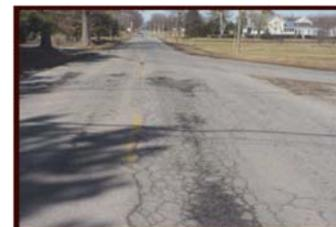
Depicts inadequate drainage and base, which results in alligatoring and rutting.
