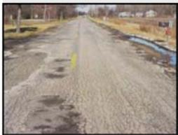
Road in Monroe County—depicts inadequate drainage. Water on roadway promotes damage (freezing and thawing).
