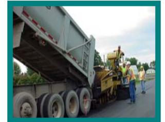
After the gravel base has been leveled, asphalt is laid. Asphalt functions like a roof over a strong gravel base. Asphalt pavement is usually laid in layers until the proper depth is achieved. That is why it seems to take so long because the crews must give one layer a chance to set before the next layer is applied. The base layer is a leveling course, the top layer is a wearing course. The
