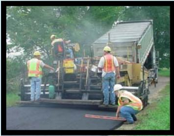
When the paving is done the restoration work is completed to help keep the water (potential ice in winter) off the road. The work of reseeding the right of way and grading the shoulders to drain the water off the roadway is extremely important.
